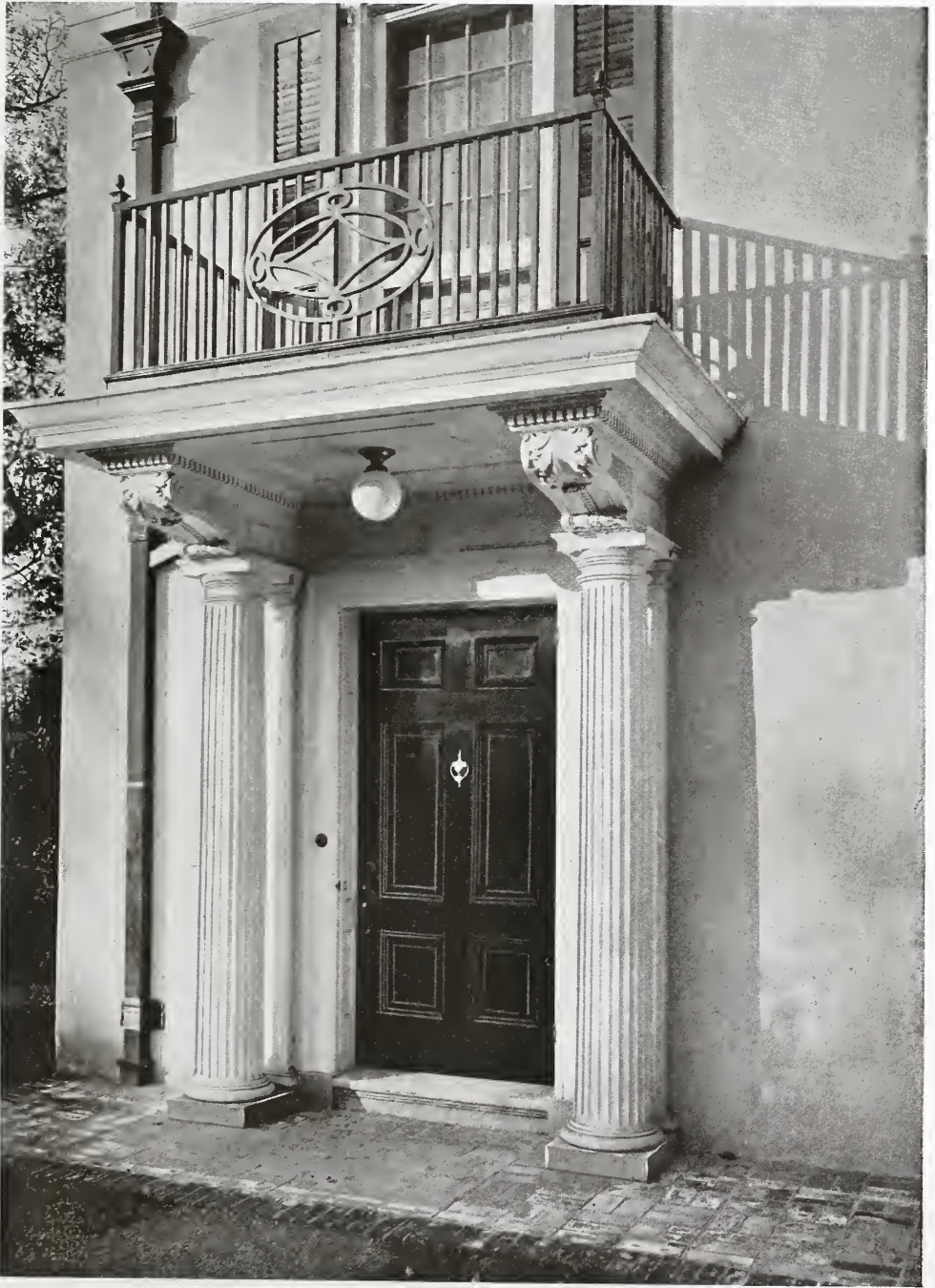
FRONT DOOR DETAIL—THE RESIDENCE OF EDWARD F. BEALE, ESQ. Stafford, Pa. Mellor & Meigs, Architects.
